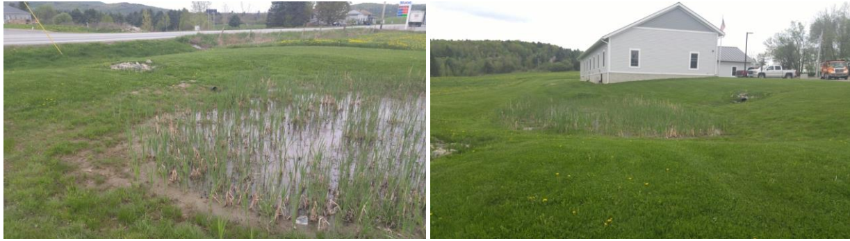
Figure 8: The current wet basin at the Town Office is proposed to be expanded and redesigned as a surface sand filter, allowing improved treatment for more runoff including from the ditches on Buck Hollow Road. The Water Quality volume (WQv) and Channel Protection volume (CPv) would be managed.
