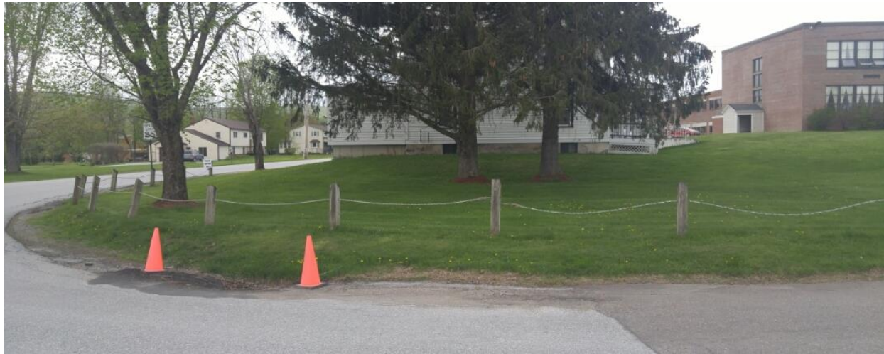
Figure 7. Stormwater infrastructure at the corner of Hunt and Maple Street is subject to excessive flow. Underground chambers placed beneath the grassy area will treat the WQv for improved management.
